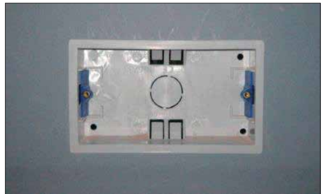
Switch box before installation of Putty Pad.
