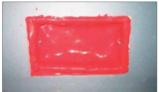
Putty Pad installed inside switch box.
